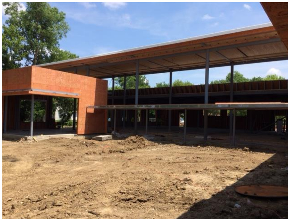
Project Site on July 3, 2018
