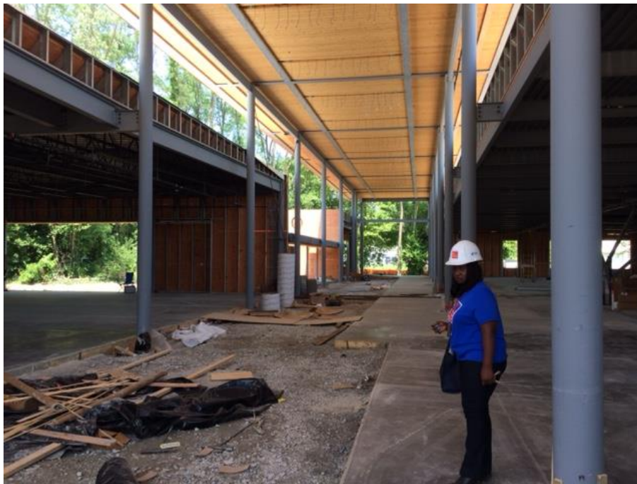
Project Site on July 3, 2018
