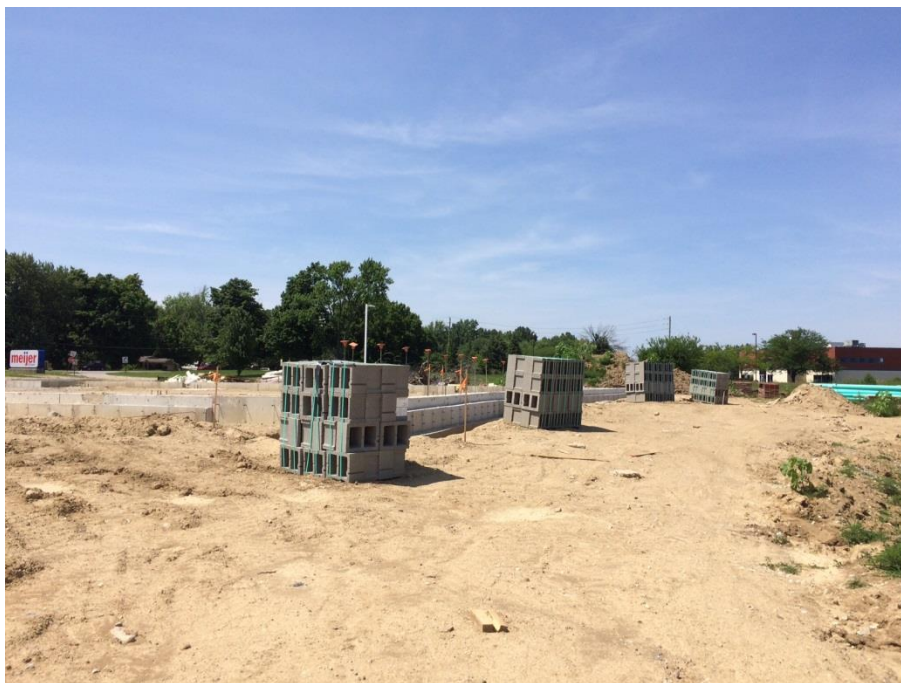
Project Site on July 11, 2018
