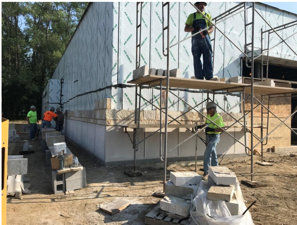
Project Site on July 12, 2018
