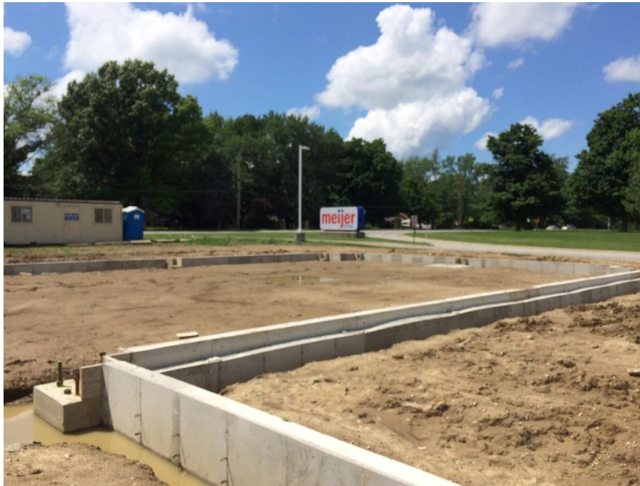
Project Site on June 26, 2018
