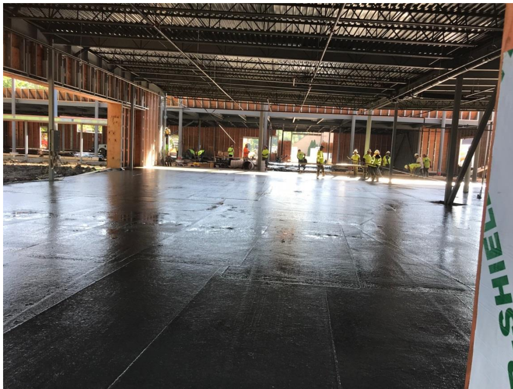
Project Site on June 28, 2018
