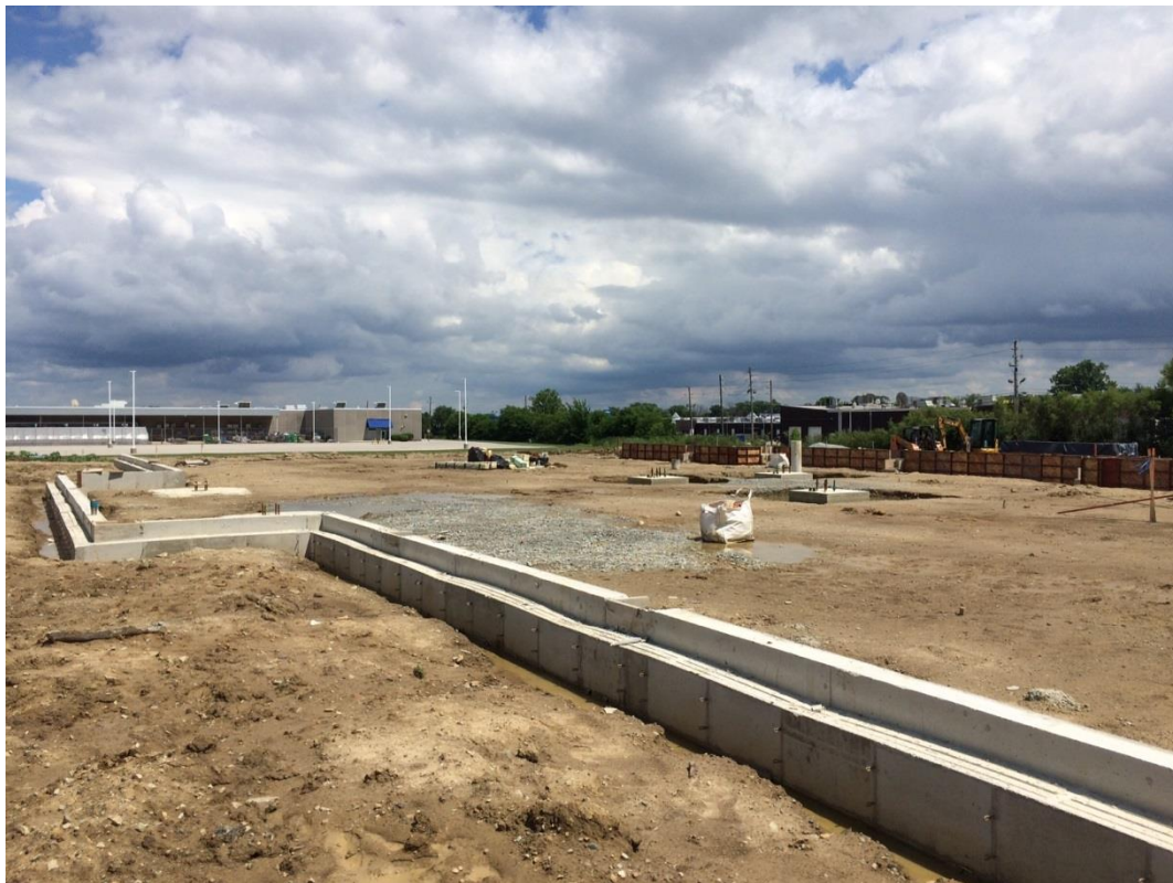
Project Site on June 26, 2018
