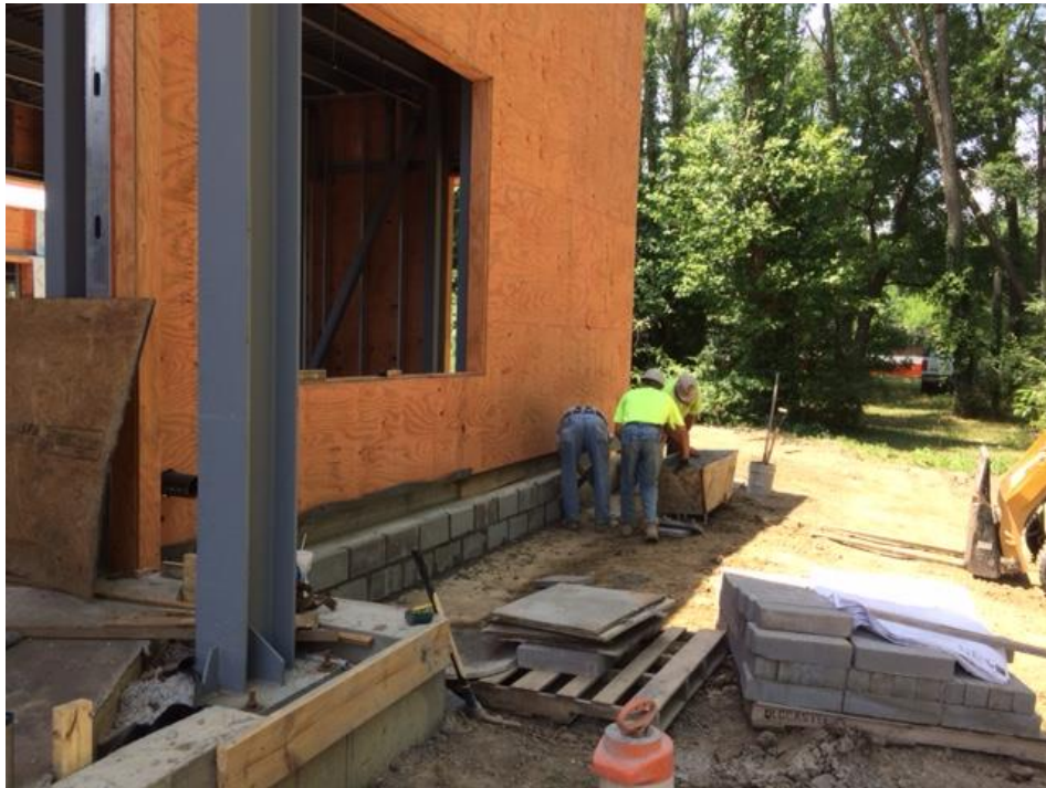
Project Site on July 3, 2018
