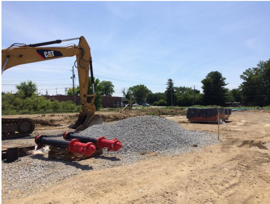
Project Site on July 11, 2018 View looking southwest showing parking area and new fire hydrants.
