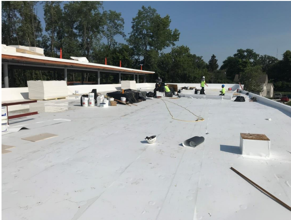
Project Site on July 12, 2018 Roofers working on the east side low roof.
